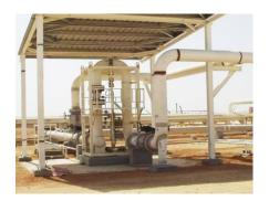
Bulk meters are large size Multiphase flow meters with sizes ranging up to 24 Inch with measurement capability of up to 500,000 BPD.
